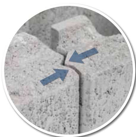
Interlocking tongue and groove joints
